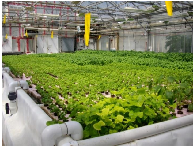
Figure 6: Basil and other plants growing in the DWC system in the CDC South Aquaponics greenhouse in Brooks, Alberta ( https://commons.wikimedia.org/wiki/File:CDC_South_Aquaponics_Raft_Tank_1_2010-07.jpg )
