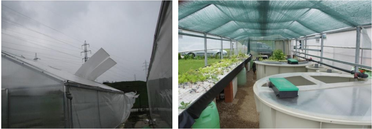
Figure 1: (left) Wind damage on a greenhouse; (b) Shading nets in a greenhouse provide protection from strong sunlight and prevent algae growth (photos: U. Strniša)
